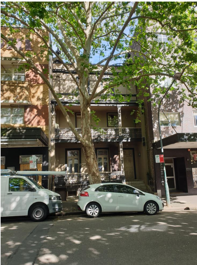
Figure 4: The former Golden Apple building viewed from Victoria St, facing west
