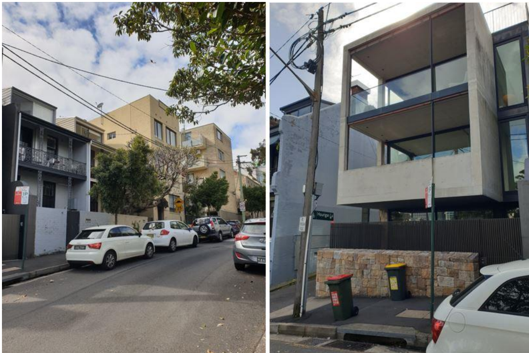
Figures 13 & 14: Terraces at 92, 94 and 98 Brougham St and residential flat building at 96 Brougham St, viewed from Brougham St facing south-east (left), and the existing development to the north of the site at 90 Brougham St, viewed from Brougham St facing east (right)
