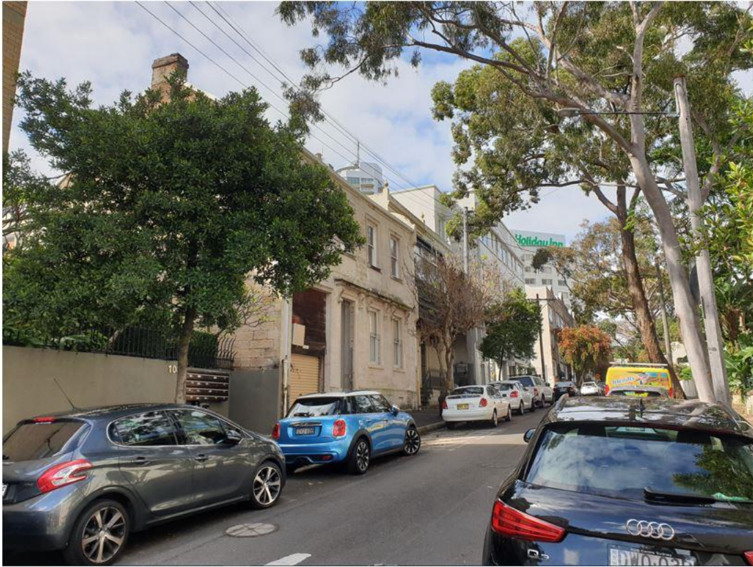
Figure 18: Existing development to the south of the site viewed from Brougham St, facing south-east
